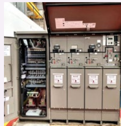
Distribution Automation Enabled Ring Main Unit (RMU)
